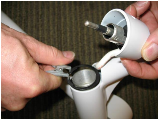
Install Spring Clip using tool
